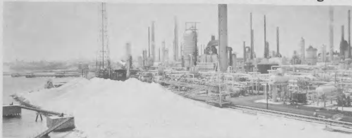
In foreground a huge pile of yellow sulfur, with HDS complex in background. Mas padilanti un monton grandi di azufre geel, cu complex di HDS banda patras.
